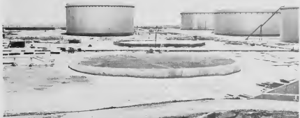
LOOKING LIKE a splattered lime in the aerial view above is an old spheroid, one of the many of this design currently being dismantled and replaced by the standard, familiar tank. Foundations for the replacement storage tanks take shape, above.
